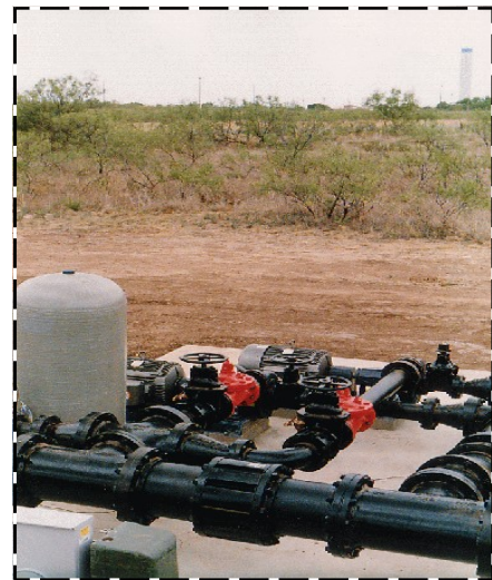
86 gallon tank replaces 30,000 gal standpipe
